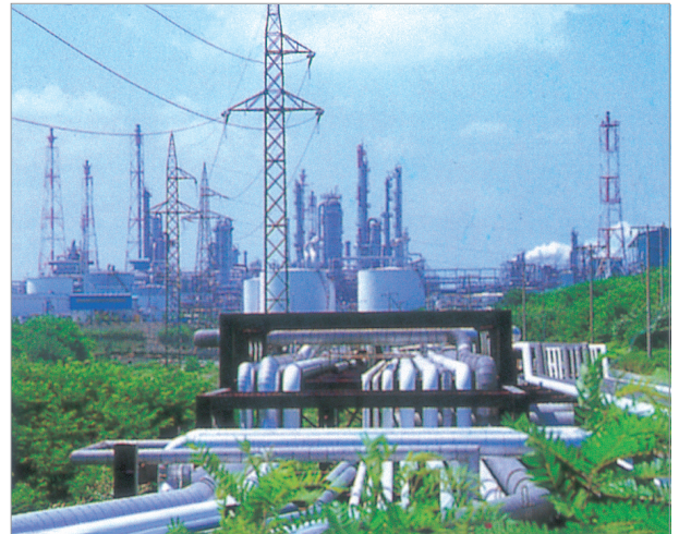
방식대상물(화학플랜트) Protected Structure(Chemical Plant)
