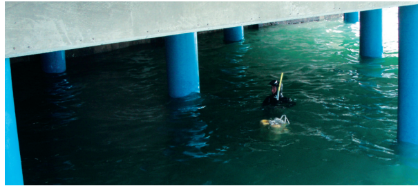
FRP 커버 설치/ Installation of FRP Cover
