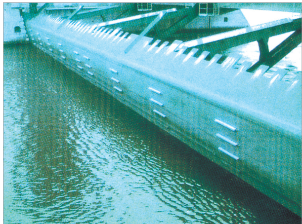
수문에 설치된 ZANODE / ZANODE Installed on Water Gate
