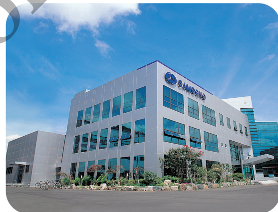
본관 전경 / View of Administration Bldg.
