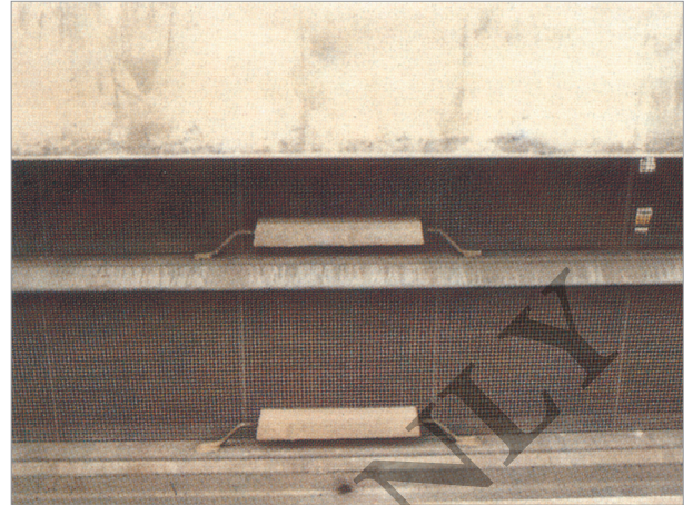
발전소 Travelling Screen용 ALUNODE / ALUNODE on Travelling Screen
