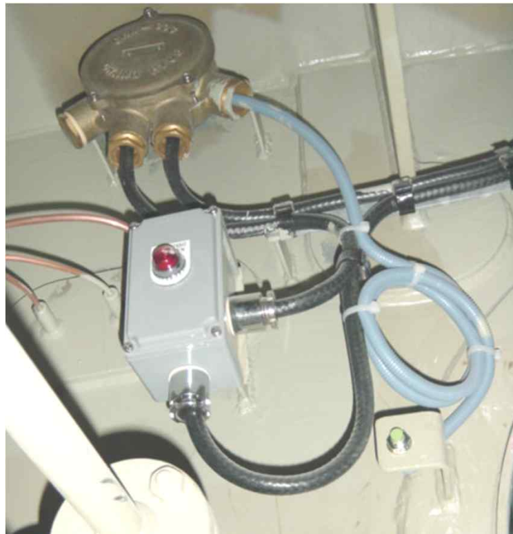
Yard에 결선된 Proximity Switch, Local Indication Box, Junction Box
