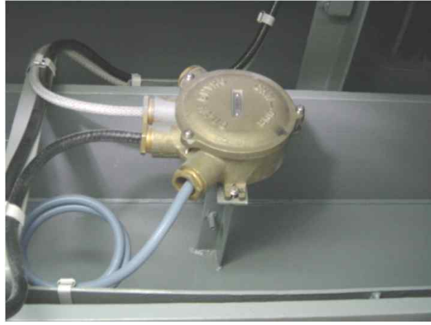
Yard에 결선된 Proximity Switch, Local Indication Box, Junction Box
