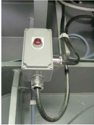
Yard에 결선된 Proximity Switch, Local Indication Box, Junction Box
