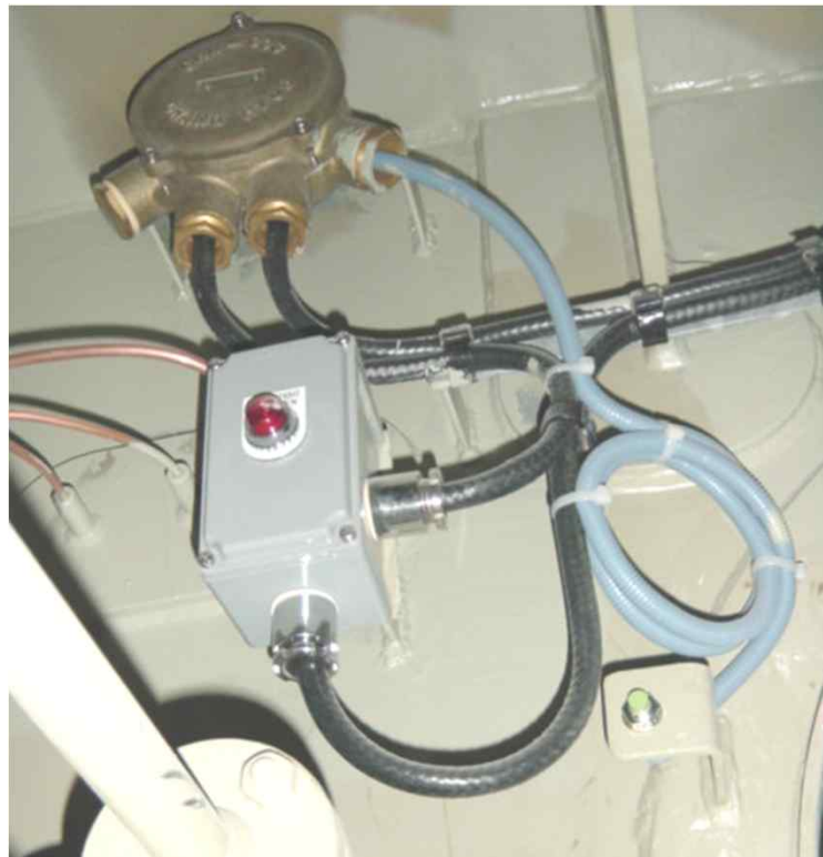
Proximity Switch, Local Indication Box and Junction Box Connected to Yard
