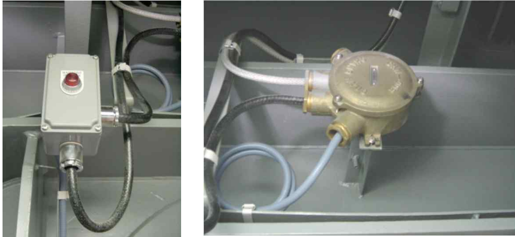
Proximity Switch, Local Indication Box and Junction Box Connected to Yard
