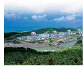
Emergency GenSets for Nuclear Power Plant
