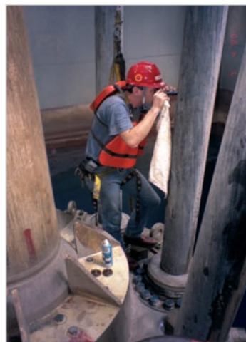
Schadensbegutachtung an Kolbenstange Damage assessment on piston rod
