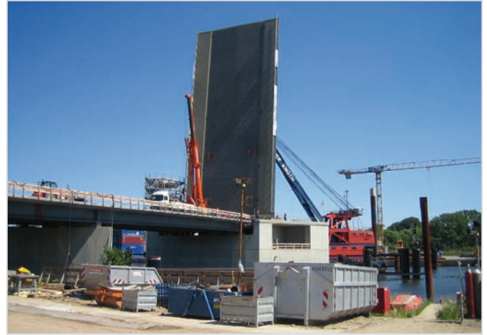
Installation of the hydraulic cylinders for the bascule bridge Lübeck, Germany
